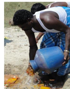
*The bricks are placed in a hole and water poured on*
